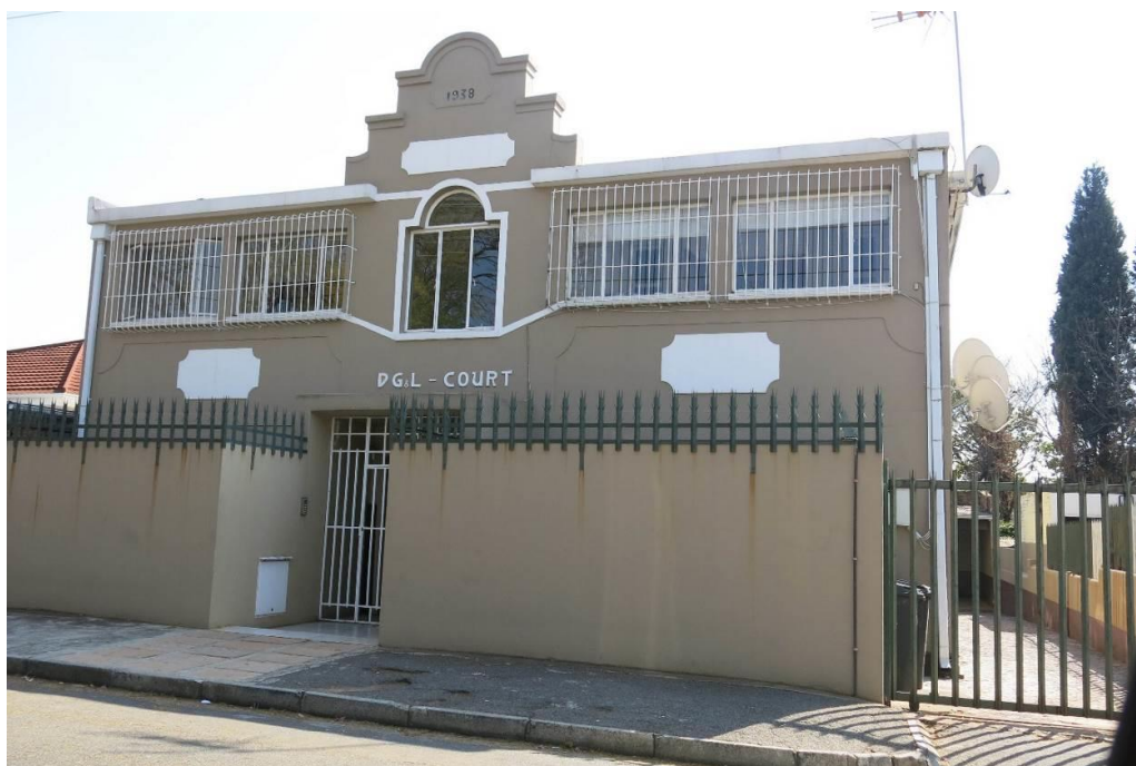
Fig. 144 Double storey apartment building with enclosed balconies on first floor level and centrally located decorative gable (Source: tsica heritage consultants, 2015)
