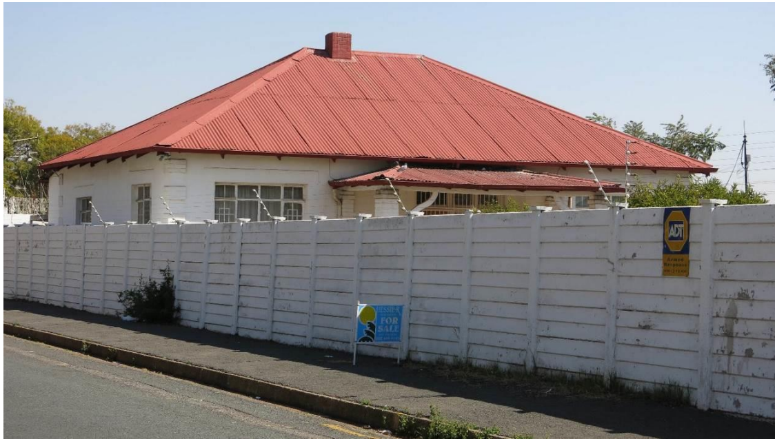
Fig. 141 Single storey freestanding residence with corrugated iron roofing and centrally located front stoep with main entrance, building corners are accentuated with corner stones and steep roof is supported with painted brick pillars (Source: tsica heritage consultants, 2015)
