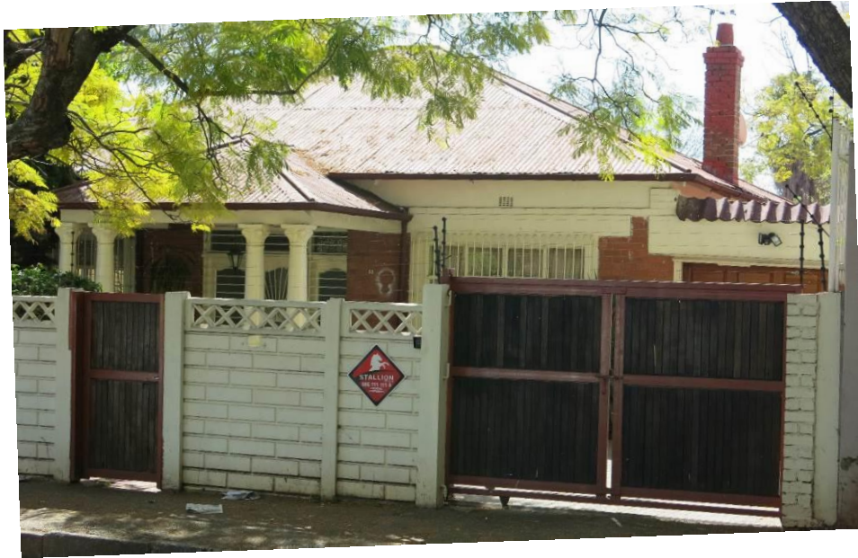
Fig. 173 Good example of single storey corrugated iron roof freestanding residence from 1933 with centrally located stoep and two sets of double columns to support the front stoep (Source: tsica heritage consultants, 2015)
