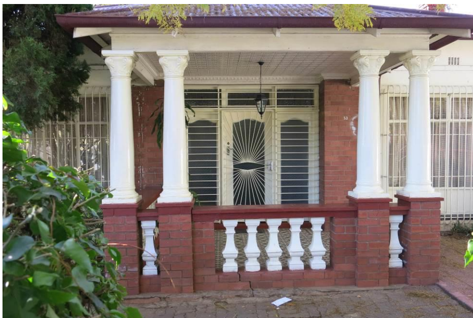
Fig. 174 Good example of a well-designed main entrance stoep with original tiling still in place (Source: tsica heritage consultants, 2015)
