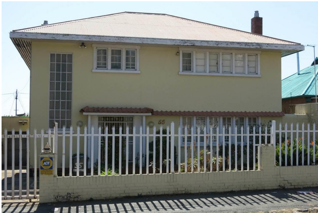
Fig. 163 Good example of double storey corrugated iron low pitched roof freestanding residence from the late 1930's with wide roof overhang and horizontal and vertical window openings (Source: tsica heritage consultants, 2015)
