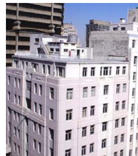
Top: photo taken from the third Corner House . Bottom left: shown in this photo (also taken from the third Corner House ), are the Lift Motor Room and Staff Quarters on the flat, concrete roof of the Clegg House – an interesting and valuable record of one of the City's 'Locations in the sky', dating from the 1930s.
