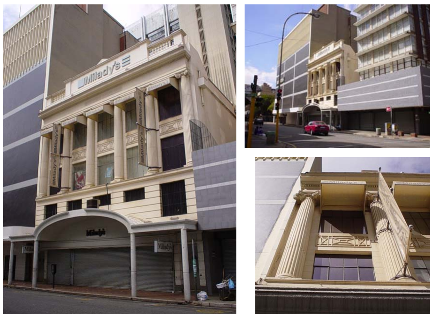
Main photo: view of main (President Street) façade. Top right: Top right: from left to right – Truworths Building, Milady's Building and City Centre.
