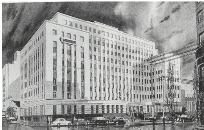
Above: Perspective of the building, c.1960, by G.A. Campbell (From Chipkin, C.M.: Johannesburg Style; Architecture & Society 1880s-1960s).
