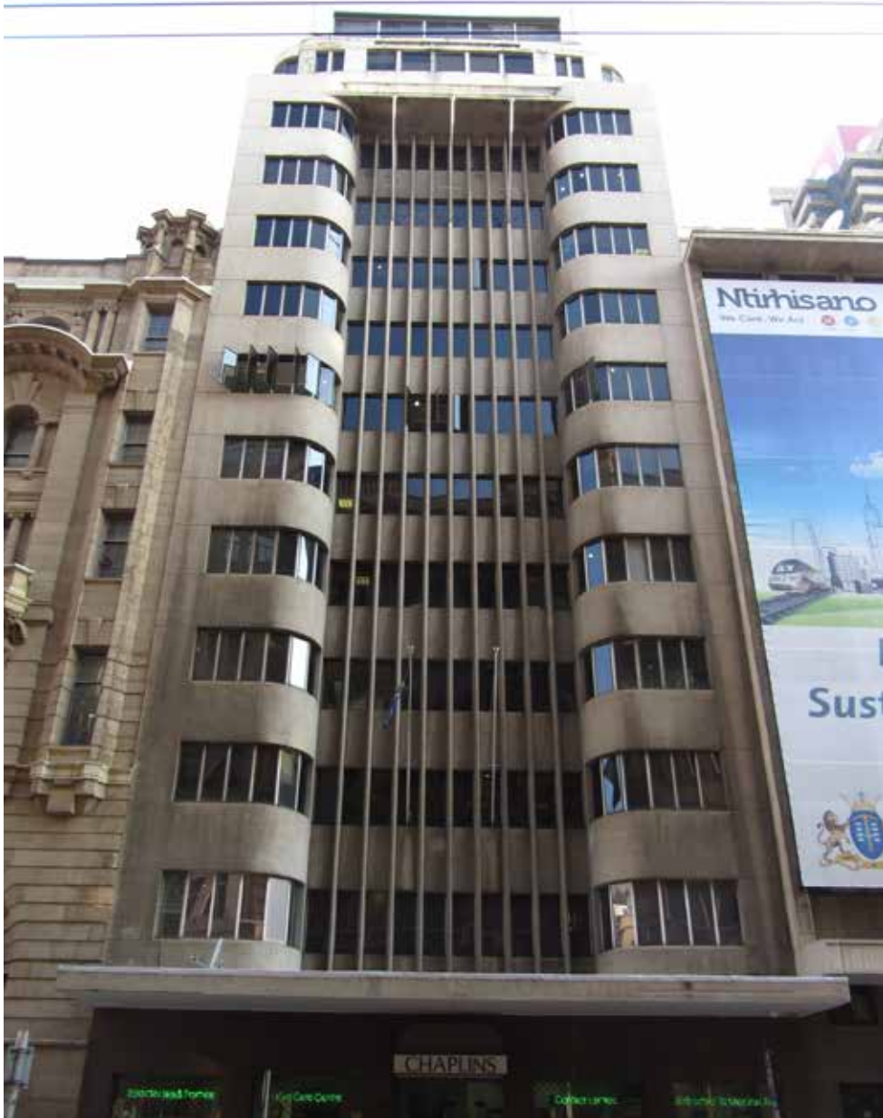
Contemporary image - facade.
