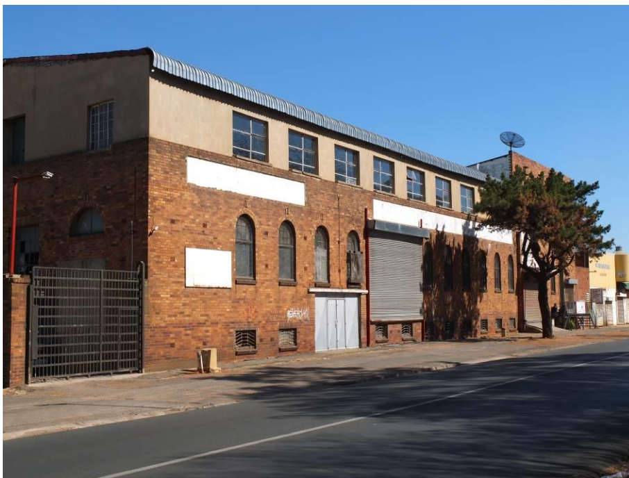
Section of original face brick workshop with line of arched windows (tsica heritage consultants, 2015)
