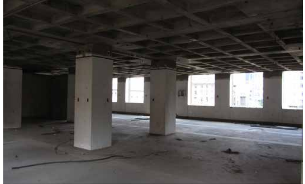
Current image - interior of upper floor.
