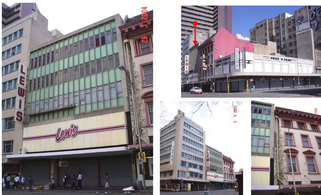
Bottom centre: from left to right – Jutas Corner Building, Lewis Building, and Geen & Richards House. Bottom right: seen in this photo is the damage caused to the façade of the Geen & Richards House due to a leaking rain collector.
