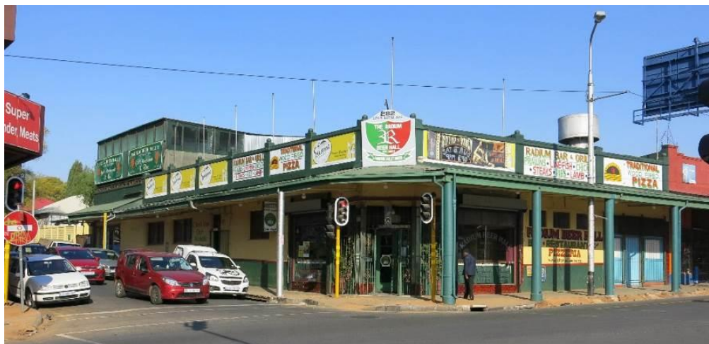
Fig. 56 Radium Beer Hall on the Corner of Louis Botha Avenue and Ninth Street (Source: tsica heritage consultants, 2015)
