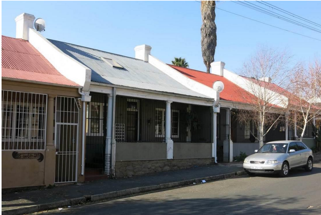
Fig. 133 Attached row houses along the northern side of 6 th Street with corrugated iron roofing and front stoeps along the sidewalk (Source: tsica heritage consultants, 2015)
