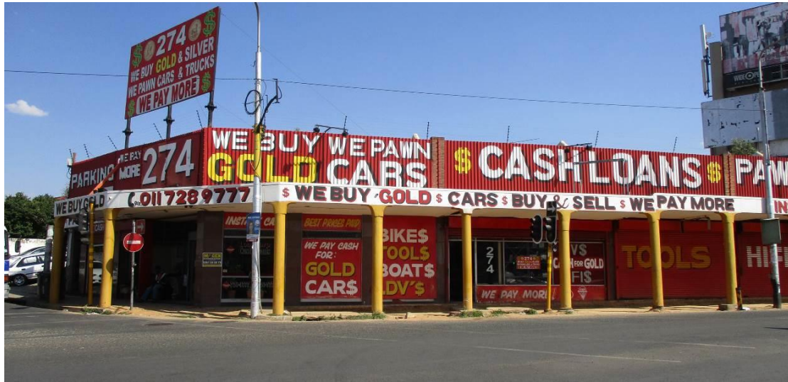
Fig. 45 Originally single storey row of shops with covered veranda along shop front (Source: tsica heritage consultants, 2015)
