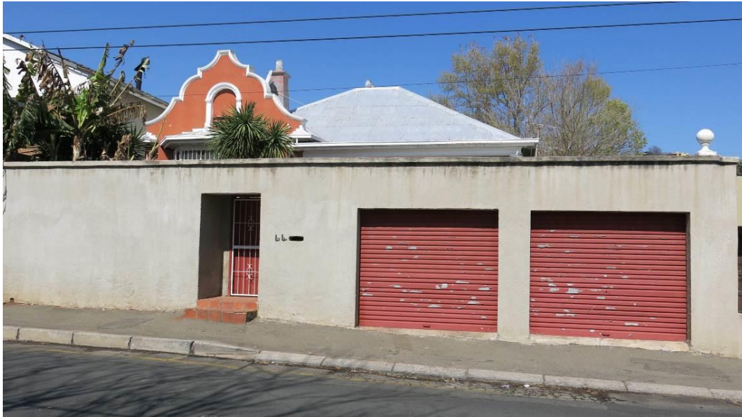
Fig. 165 Good example of single storey corrugated iron roof freestanding residence from the around 1910 with decorative front gable and stoep around the corner (Source: tsica heritage consultants, 2015)
