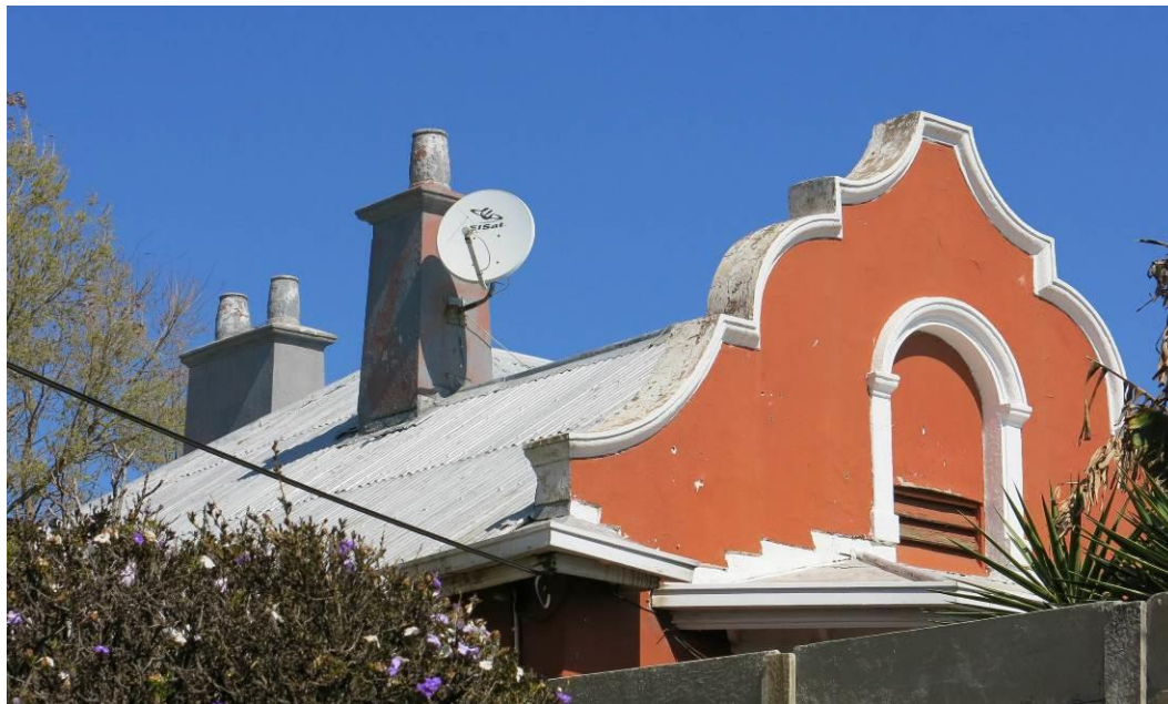
Fig. 166 Corrugated iron roof structure with chimneys and decorative gable points to elaborate architectural design from around 1910 (Research in progress) (Source: tsica heritage consultants, 2015)
