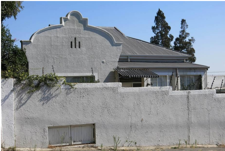
Fig. 119 Semi-dutch gabled building along the south-western side of Second Avenue, Stand 558 (Source: tsica heritage consultants, 2015)
