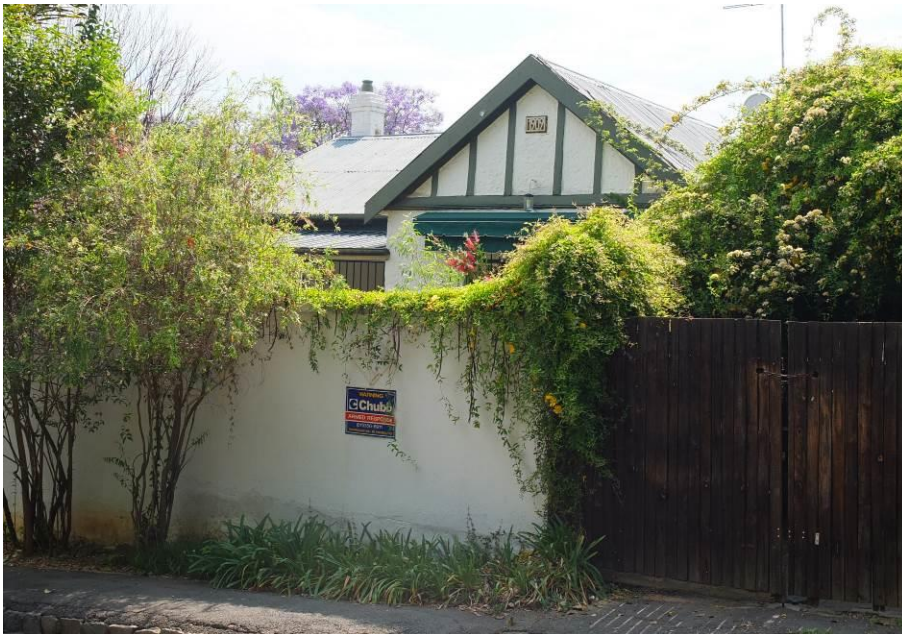
Fig. 124 One sided triangular gable with front stoep and pitched corrugated iron roofing (Source: tsica heritage consultants, 2015)
