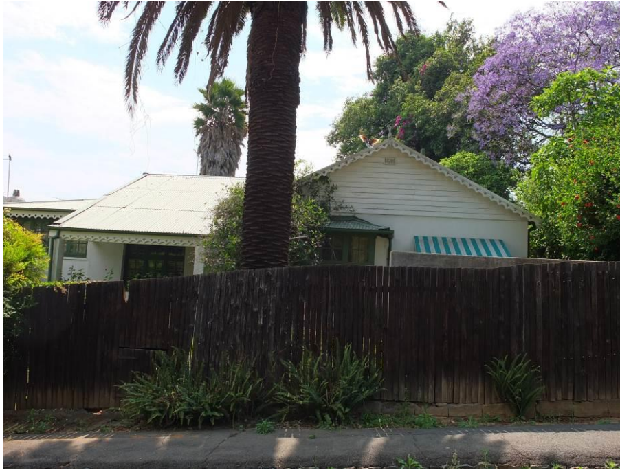
Fig. 123 One sided triangular gable with front stoep and pitched corrugated iron roofing (Source: tsica heritage consultants, 2015)
