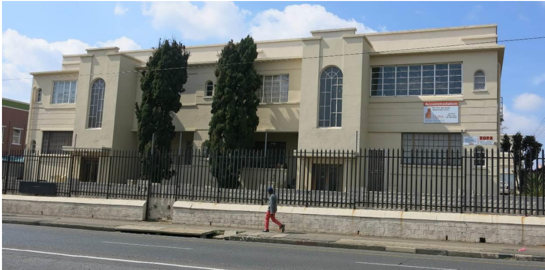
Fig. 79 East elevation along Louis Botha features two main entrances with staircase section breaking the horizontally structured façade vertically (Source: tsica heritage consultants, 2015)
