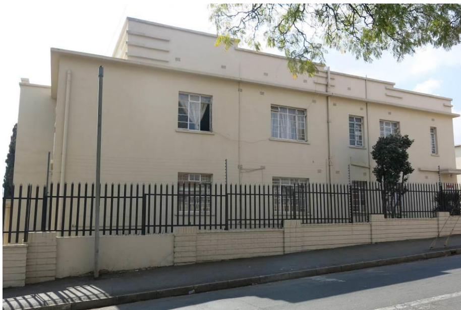
Fig. 80 South elevation along Sixteenth Street (Source: tsica heritage consultants, 2015)
