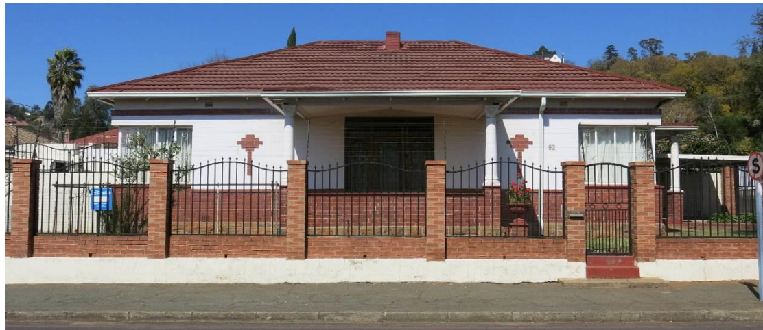
Fig. 138 The tiled roof building shows fine face brick detailing along the façades and corner windows opening the façade to the sides (Source: tsica heritage consultants, 2015)
