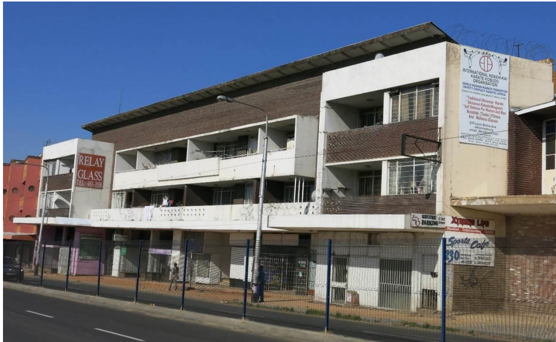
Fig. 30 Three storey commercial mixed-use building block along Louis Botha Avenue (Source: tsica heritage consultants, 2015)
