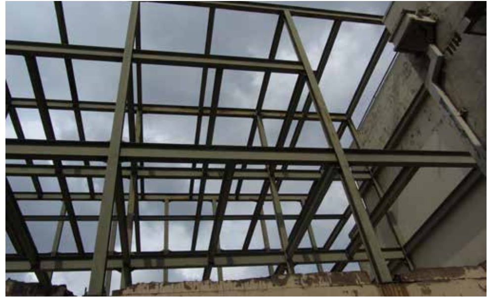
Contemporary image -detail of steel structure on roof.
