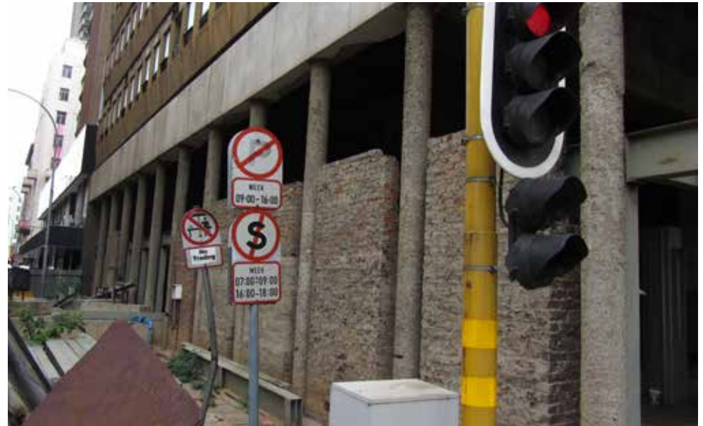
Contemporary image - bricked up Ground Floor.
