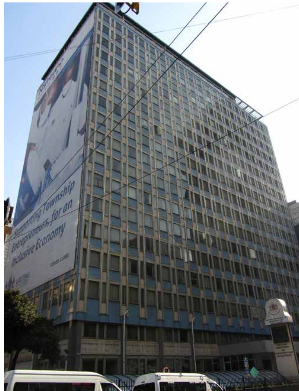
Contemporary image - exterior facade.
