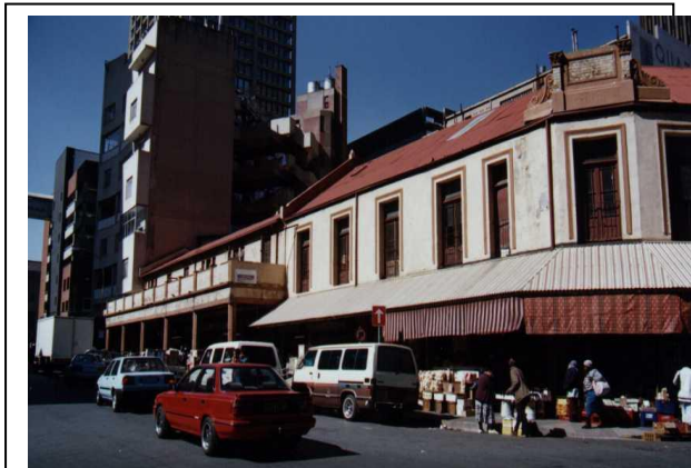
Jhb Metro - Cool Factory
