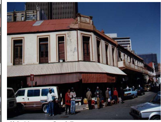
Jhb Metro - Cool Factory
