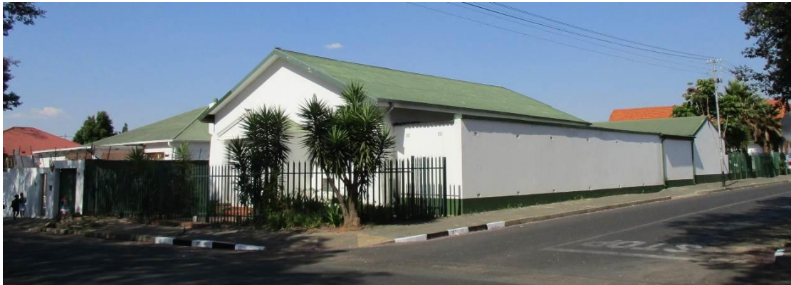
Fig. 90 Former Scout Hall from 1925 on the corner of Eighth Avenue and Thirteenth Street (Source: tsica heritage consultants, 2015)
