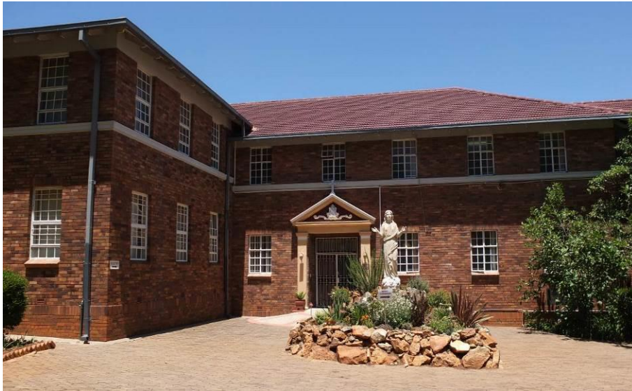
Fig. 191 School buildings consists of double storey face brick buildings with low pitched tiled roofing and classical decorative elements around the main entrance (Source: tsica heritage consultants, 2015)
