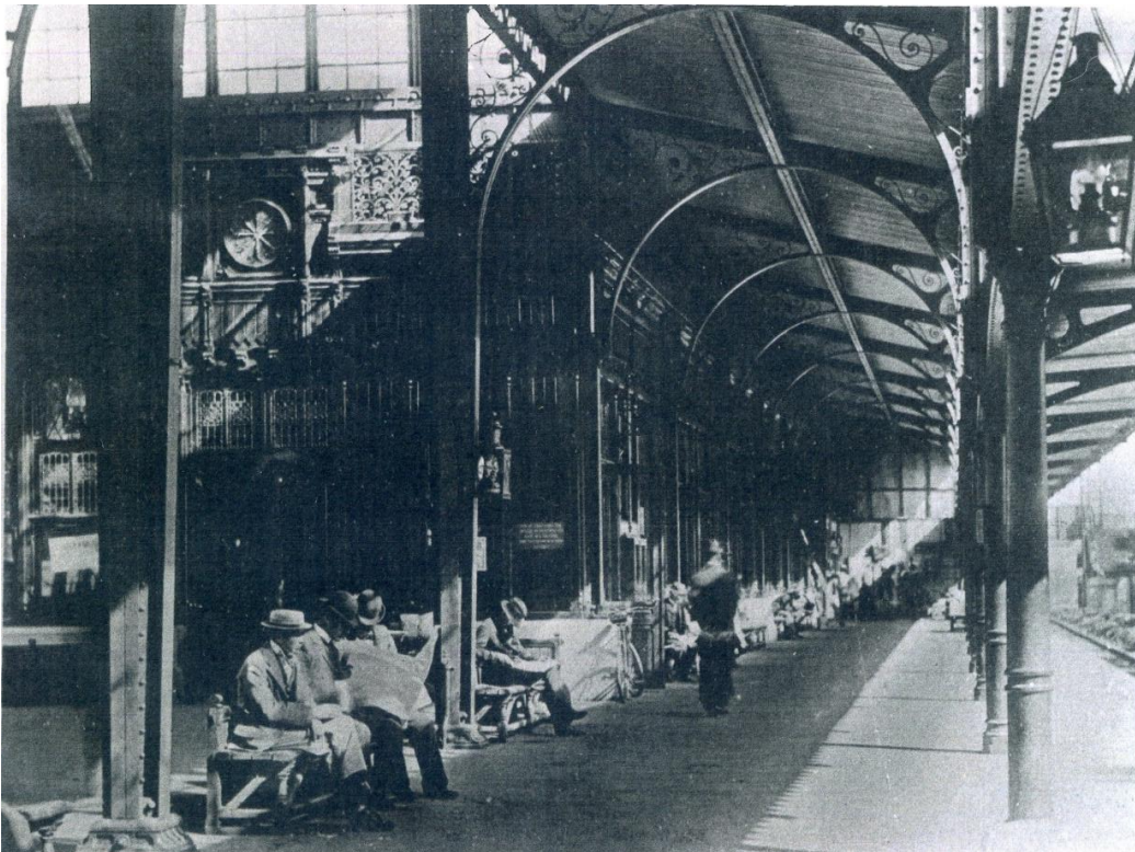
Old Park Station Interior in c.1902, note the highly ornate detailing to the timber kiosks. Museum Africa
