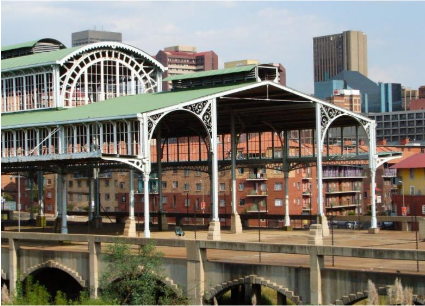
Photograph looking south, with Brickfields South visible through the structure, Panoramio website. This photograph shows the abrupt termination of the roof vent, which would have had a grille to its face
