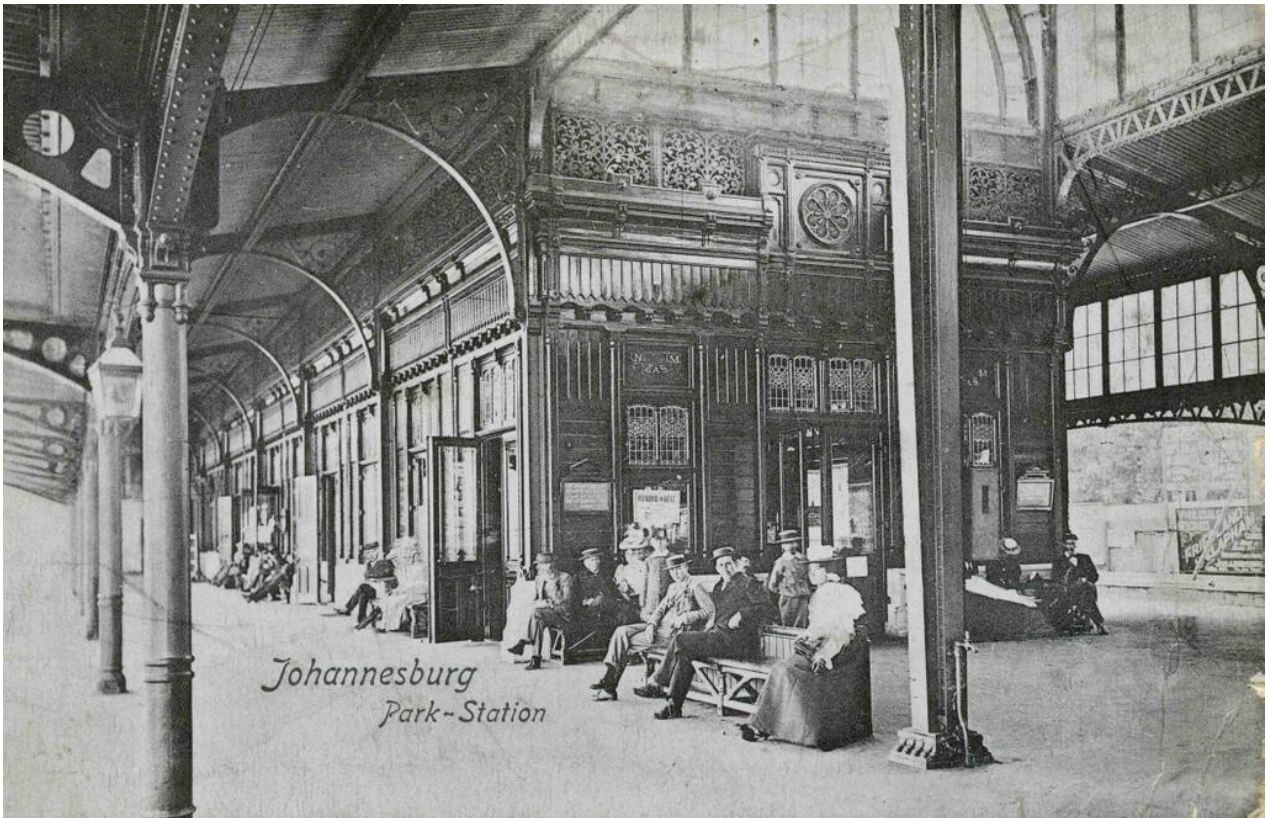
View of the principal building on the main platform of Old Park Station c.1902. The timber panelling is richly detailed with deep profiles and cornices. Above the panelling are ornate cast iron grilles. The column in the foreground shows the detailing to the cast columns and structural bracing, the rhythm of the rivets also forms part of the aesthetic. Photograph from Transnet Heritage collection.
