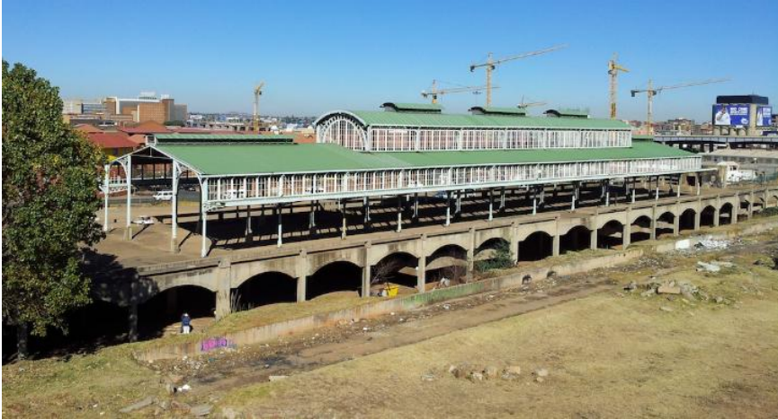
Photograph of Old Park Station c.2002 in its current location in Newtown North, during the building of Mandela Bridge, heritageportal.co.za
