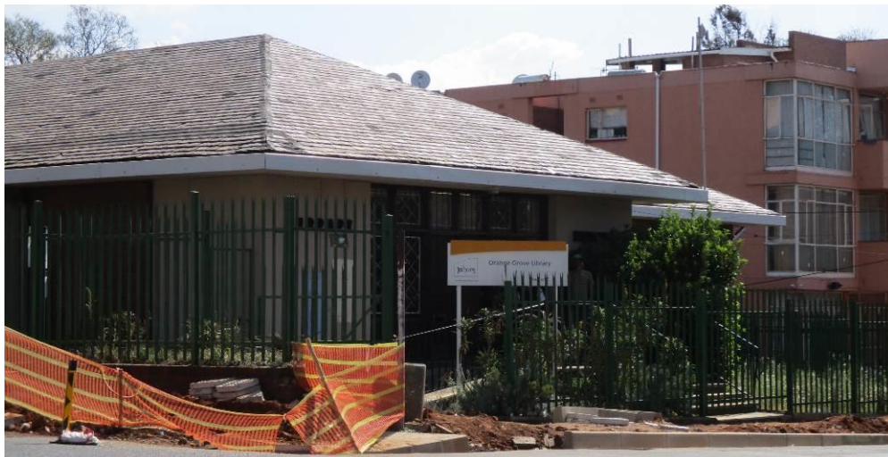
Fig. 84 Main entrance to Library along the southern side of Thirteenth Street (Source: tsica heritage consultants, 2015)
