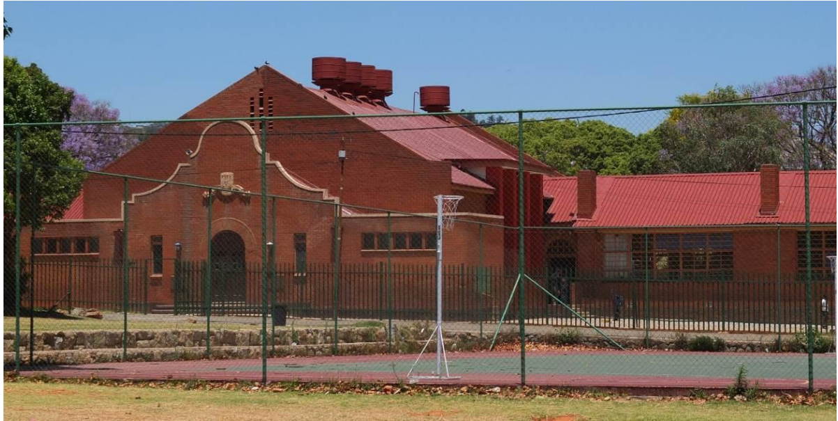
Fig. 200 School buildings consists of single storey red face brick buildings with low pitched corrugated iron roofing and with air vents and gabled entrance (Source: tsica heritage consultants, 2015)
