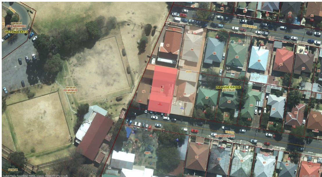
Fig. 93 Stands 52 to 55 are located along the northern side of Tenth Street, East of Paterson Park North
