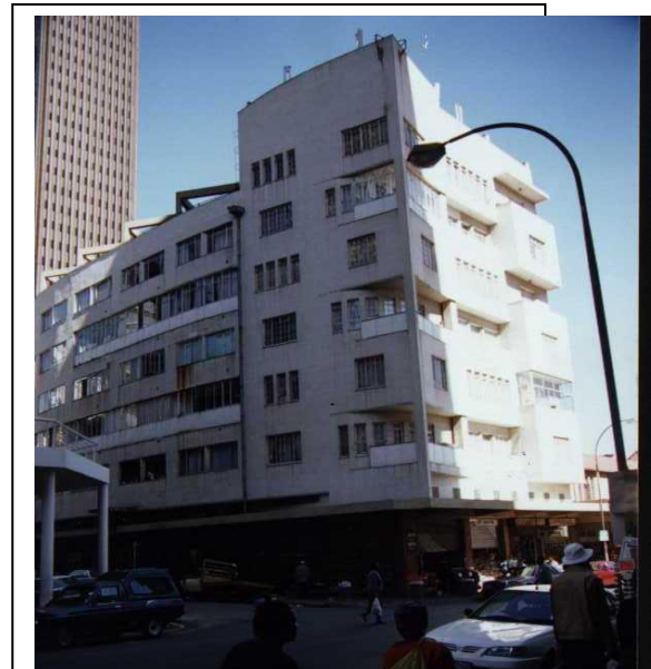
Jhb Metro - Cool Factory
