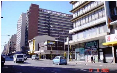
Bottom left: view of the subject building in the middle-background. Its Bree Street neighbour, the Cutler & Wilson Building , is also clearly visible in these photos.
