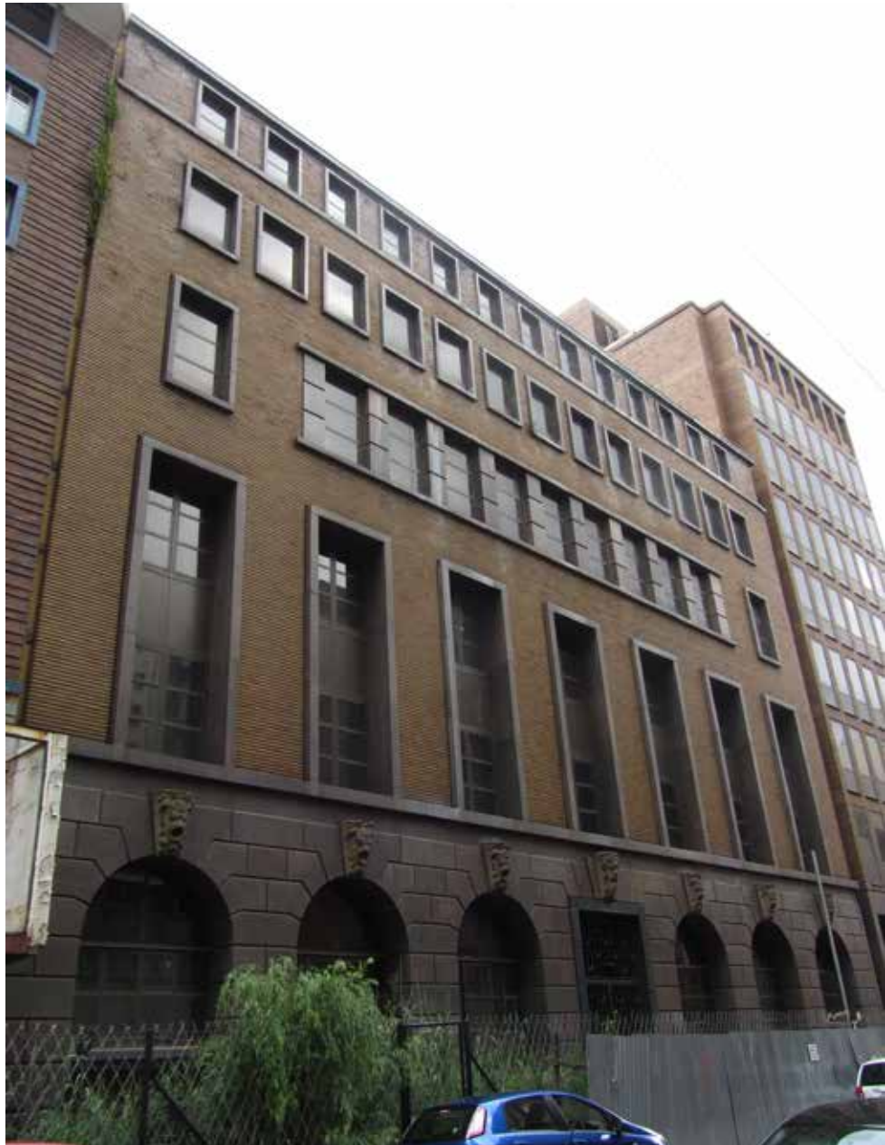
Contemporary image - facade.
