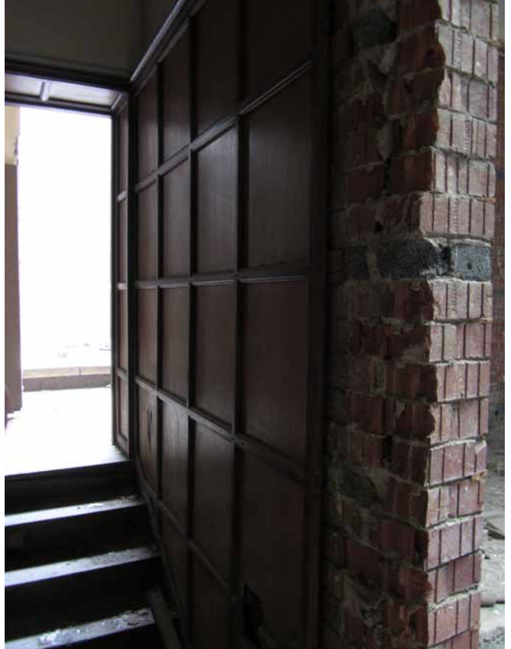
Contemporary image - interior of Ground Floor.
