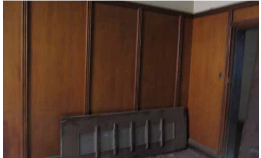
Contemporary image - interior panelling on upper floor.
