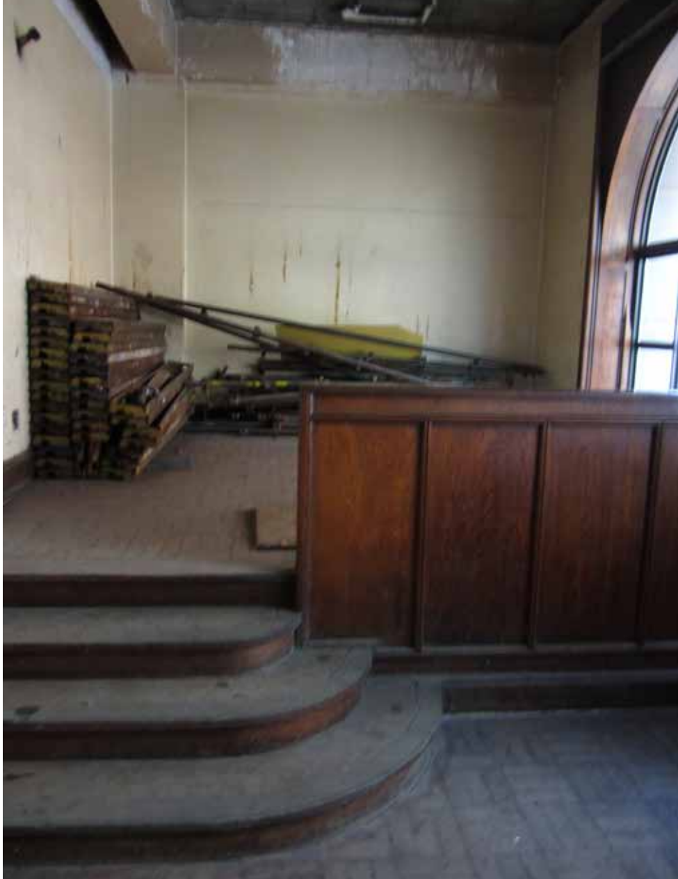
Contemporary image - interior of Ground Floor.
