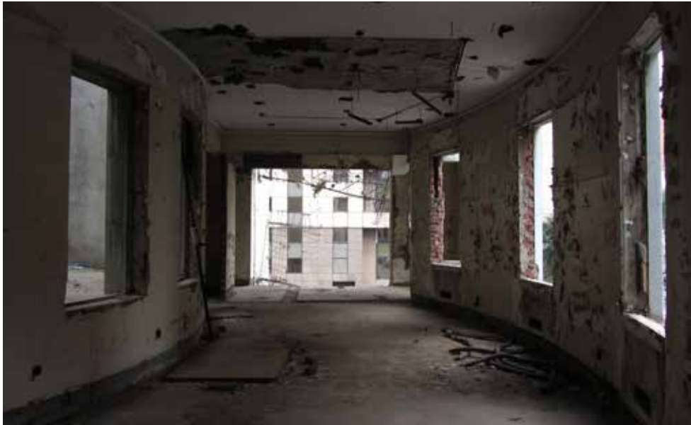
Contemporary image - interior / outer area of chamber room.
