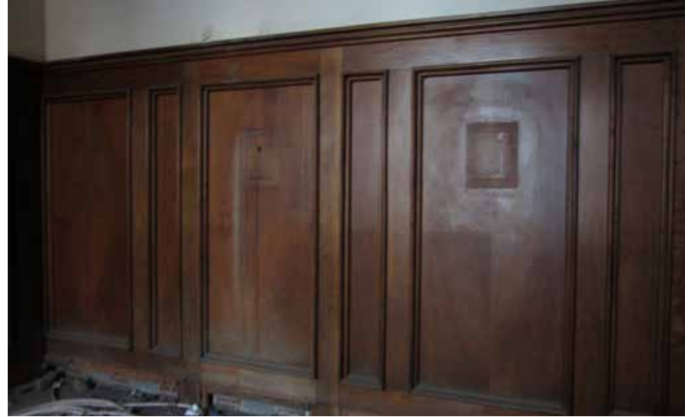
Contemporary image - interior panelling on upper floor.
