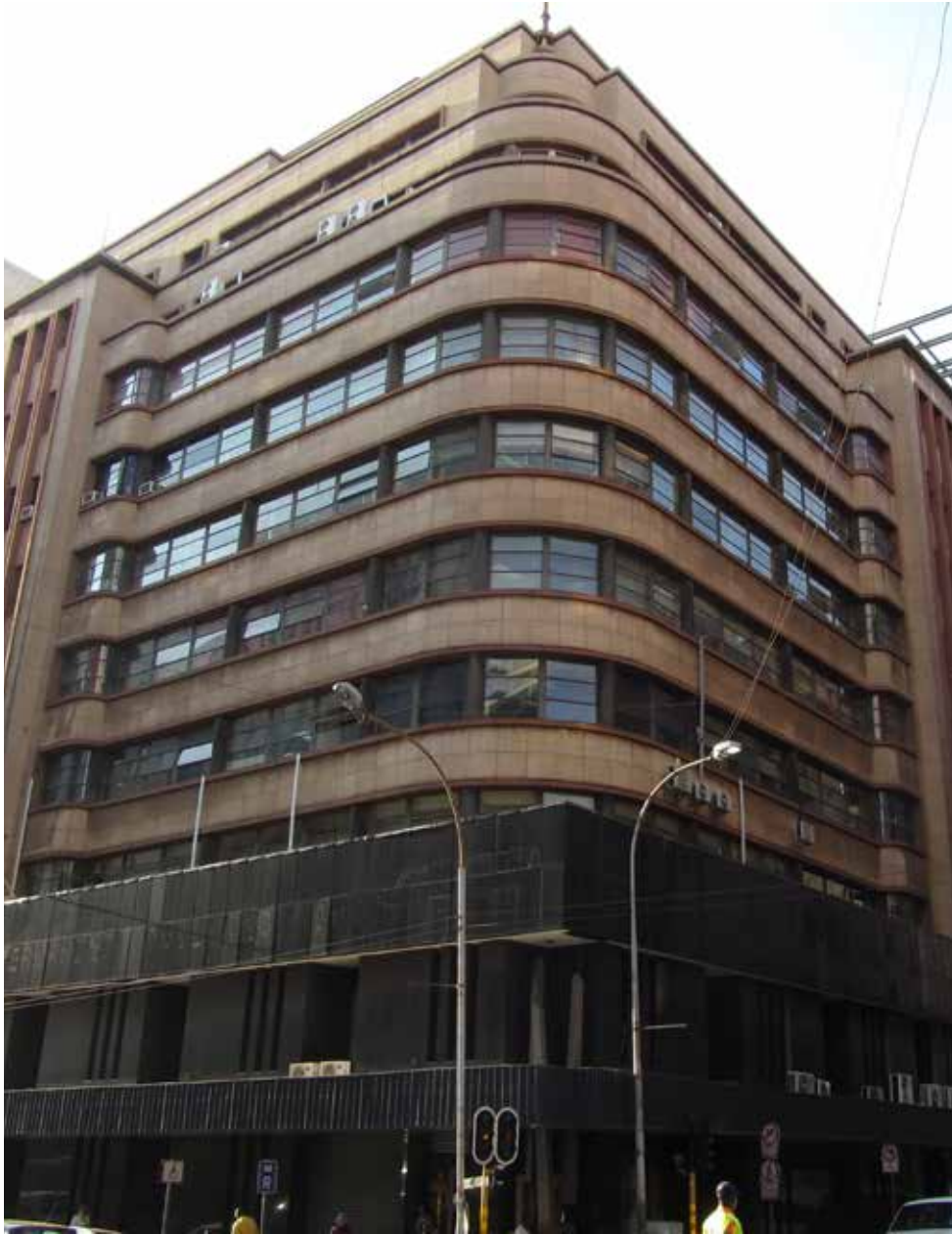
Contemporary image - corner facade of building.
