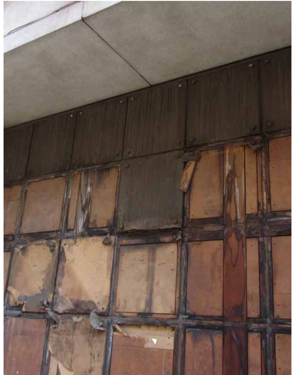
Detail of missing bronze panels on the vehicular entrance door.
