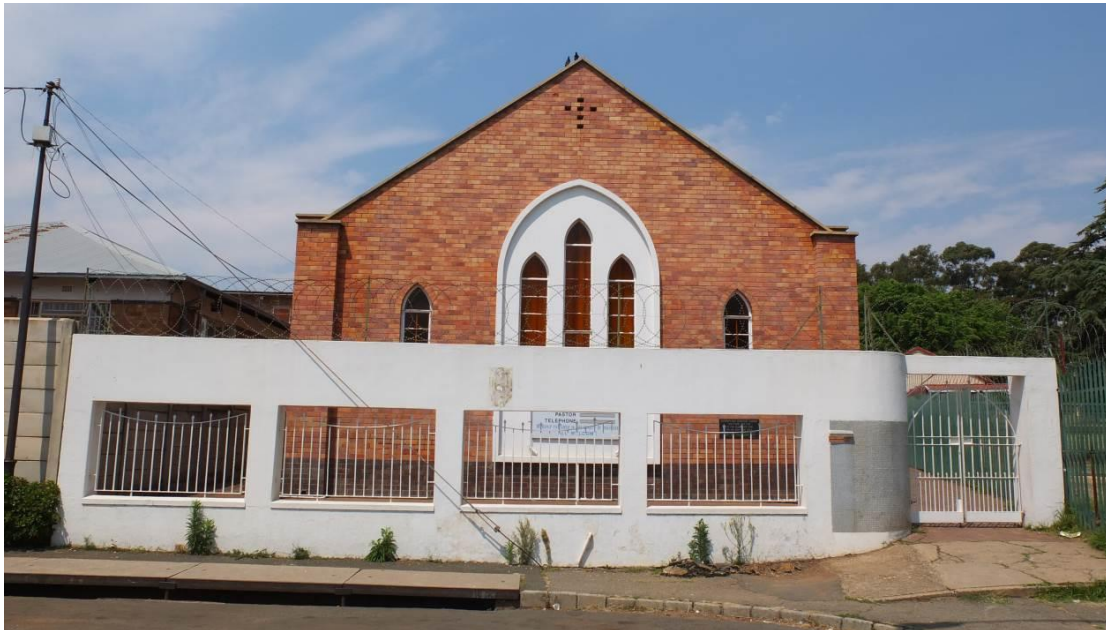
Fig. 100 Seventh Day Adventists Church with face brick façade and pointed arched long narrow windows (Source: tsica heritage consultants, 2015)
