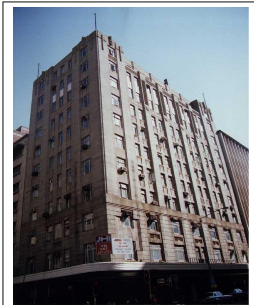
Jhb Metro - Cool Factory
