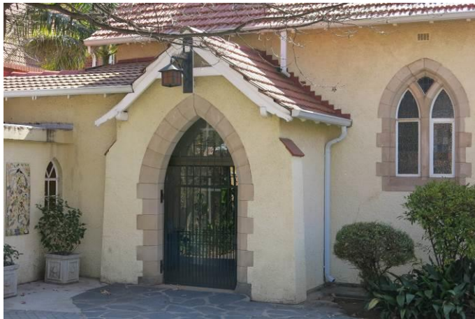
Fig. 108 Original main entrance to church by FLH Fleming (Source: tsica heritage consultants, 2015)
