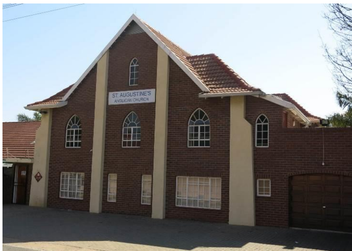
Fig. 109 Later built double storey church building (Source: tsica heritage consultants, 2015)
