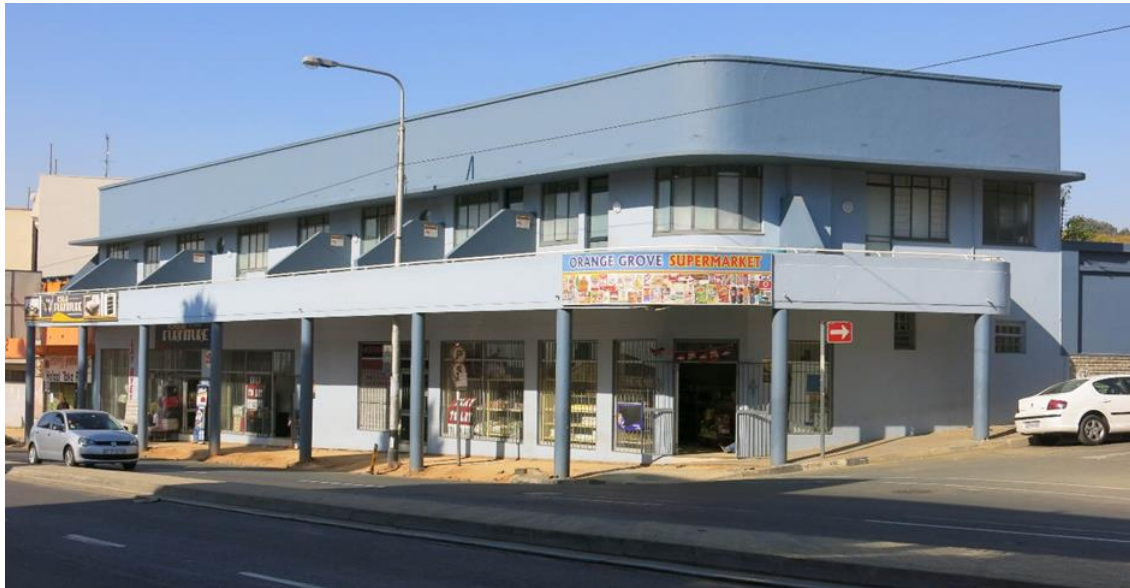
Fig. 35 Two storey commercial building with columns supported veranda along Louis Botha Avenue (Source: tsica heritage consultants, 2015)
