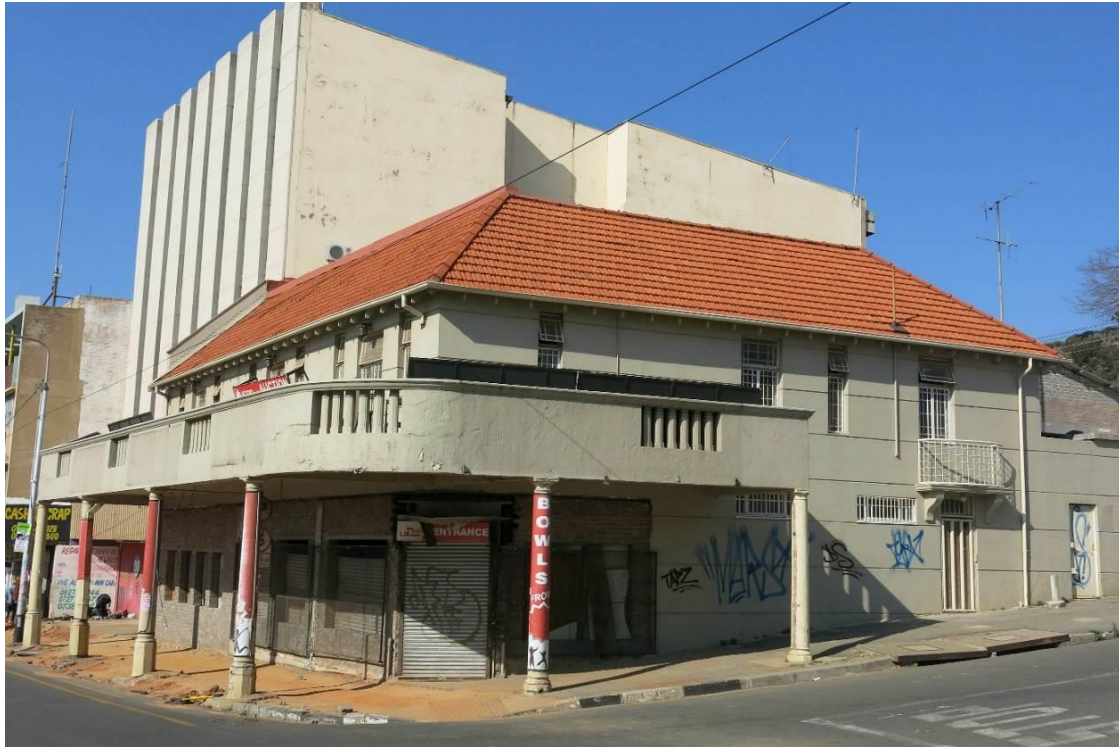
Fig. 28 Double storey building on the corner of Louis Botha Avenue and First Street (Source: tsica heritage consultants, 2015)
