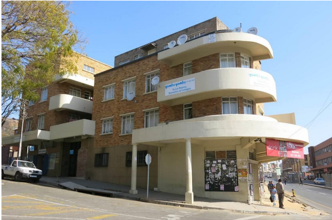
Fig. 39 Four storey commercial mixed-use building with shops on street level and apartments above along the south-western corner of Third and Louis Botha Avenue (Source: tsica heritage consultants, 2015)
