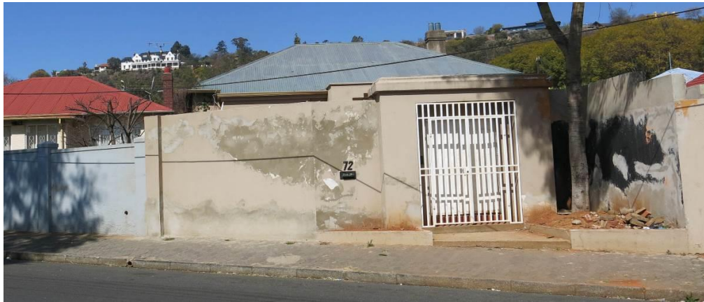
Fig. 158 Good example of three single storey corrugated iron roof freestanding residences from around 1920's with centrally located front stoep (Source: tsica heritage consultants, 2015)
