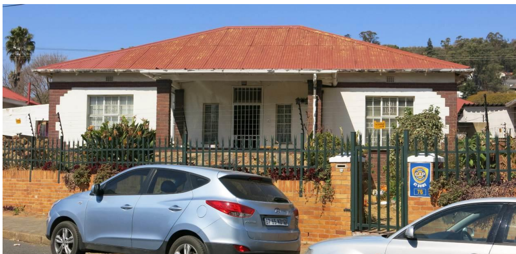
Fig. 160 Corrugated iron roof house with centrally located stoep and face brick detailing along the edges of the building (Source: tsica heritage consultants, 2015)
