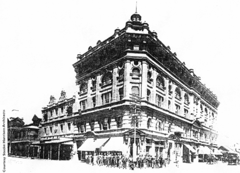
Victory House, where Johannesburg's first lift had crowds gaping for weeks
